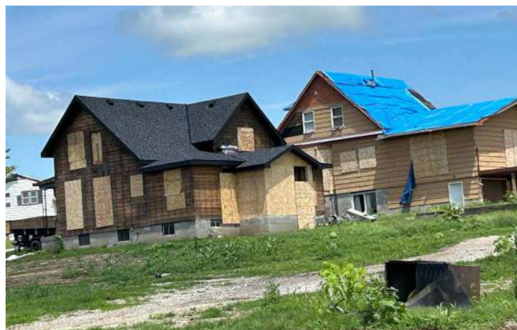
Damage caused by tornado i n Minden, Iowa
