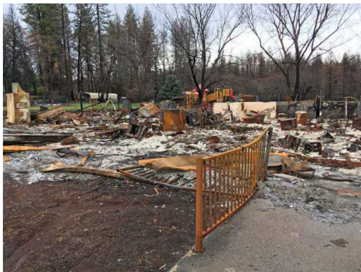
Damage caused by wi ldfires in California
